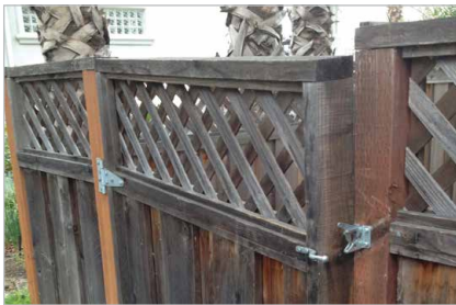
RTA2 90° ANGLE REINFORCEMENT
