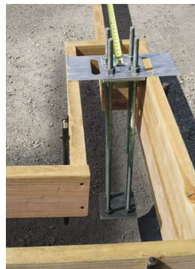
Strong Frame OMFSL anchorage assemblies make design and installation faster and easier
