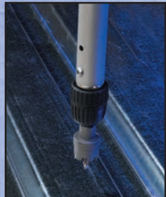
2. Drill Deck Holes
