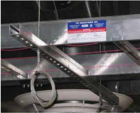
Trapeze hangers with strut
