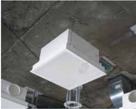
Hangers attached to brackets
