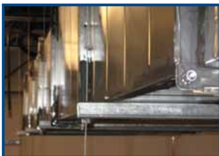
Rectangular duct with strut
