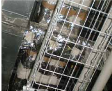
Trapeze hangers with strut
