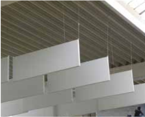
Acoustic baffle
