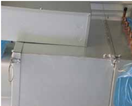
Duct trapeze hangers
