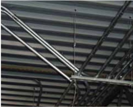
Trapeze hangers with strut
