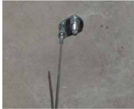
90° Eyelet in concrete
