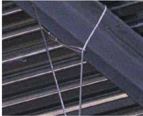
Loop choked around bar joist
