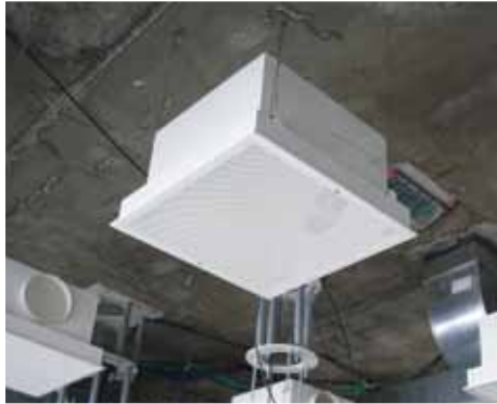
Hangers attached to brackets
