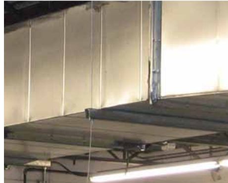
Trapeze hanger with struts
