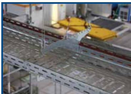
Cable tray with G-Bracket
