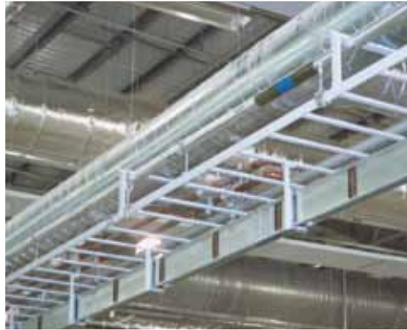
Standard Gripple HF through eyebolts
