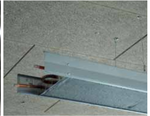
Hangers attached to unit
