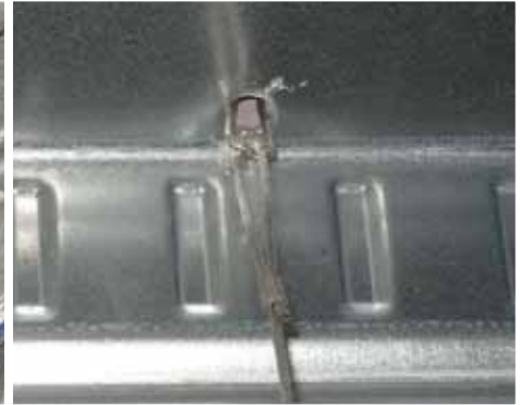
Loop with concrete wire anchor
