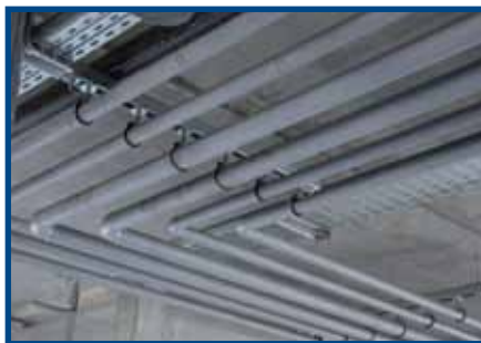
Steel pipes heating
