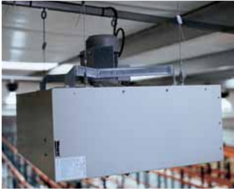
Hangers attached to unit
