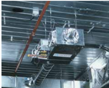
Hangers attached to unit
