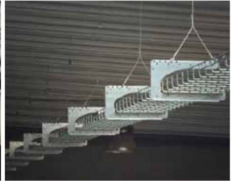
Y-Fit hanger with G-Bracket
