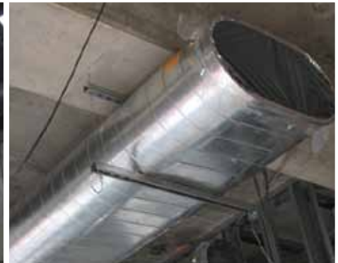
Trapeze hanger with strut
