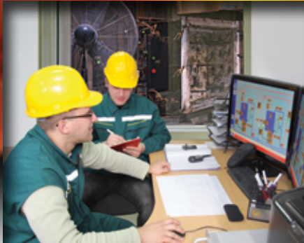
Combustion control room
