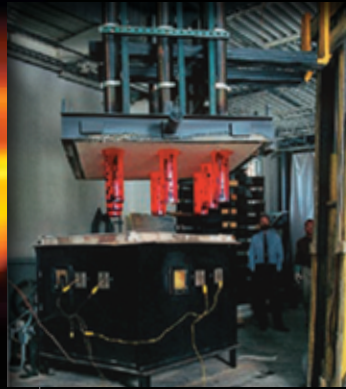
On-site test furnaces
